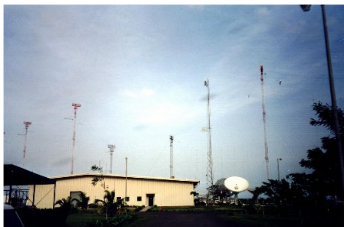
The IBB transmitter building in front of some of the SW antennas. The satellite dishes are seen to the right.
