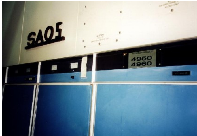
Close look at the eldest IBB transmitter on São Tomé which now is used for the 60 meter tropical band.
